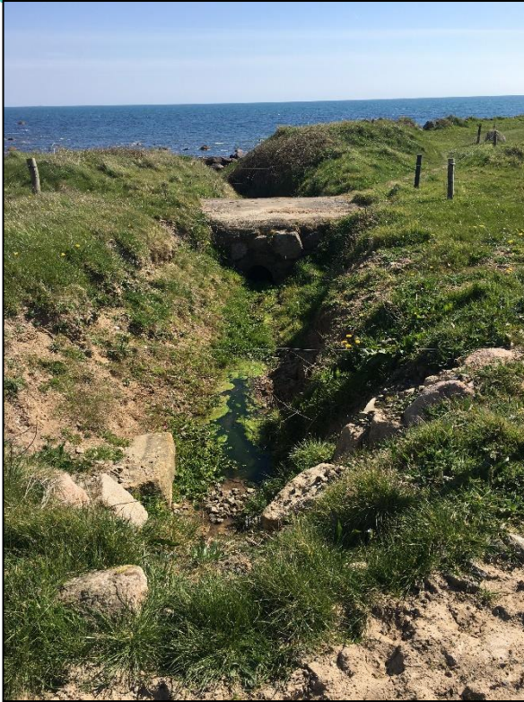
Plate 9-1 Typical drainage channel on site
